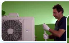
Insert the tube, previously cut and deburred, into the nut and the insert the sleeve. Bevel of sleeve toward nut. Lubricate the inner surface of the nut.
