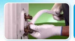
Apply pressure to hold tube against male flare body while hand tightening. Mark pipe-nut location then follow wrench tightening directions. If necessary maintain pressure on tube until nut tightening prevents tube drift.
